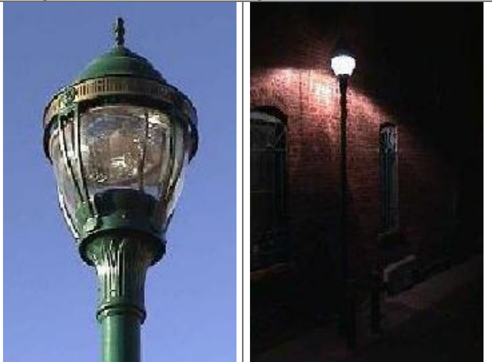
"Antique" Fixture with Recessed Lamp
